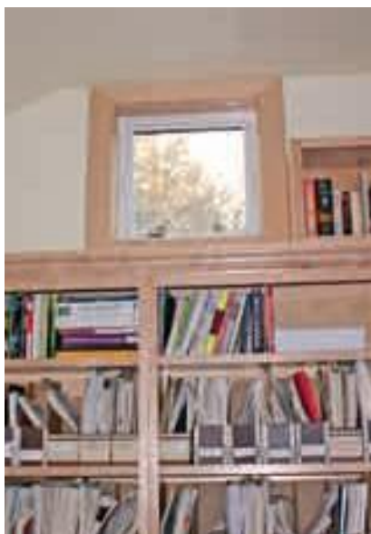
Operable windows placed high in the second-floor rooms provide ventilation using natural convection.
