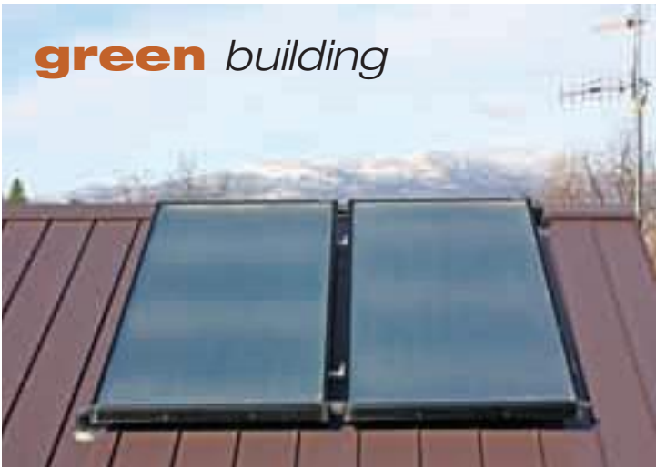
Two solar thermal collectors offset 68% of water-heating energy loads.
